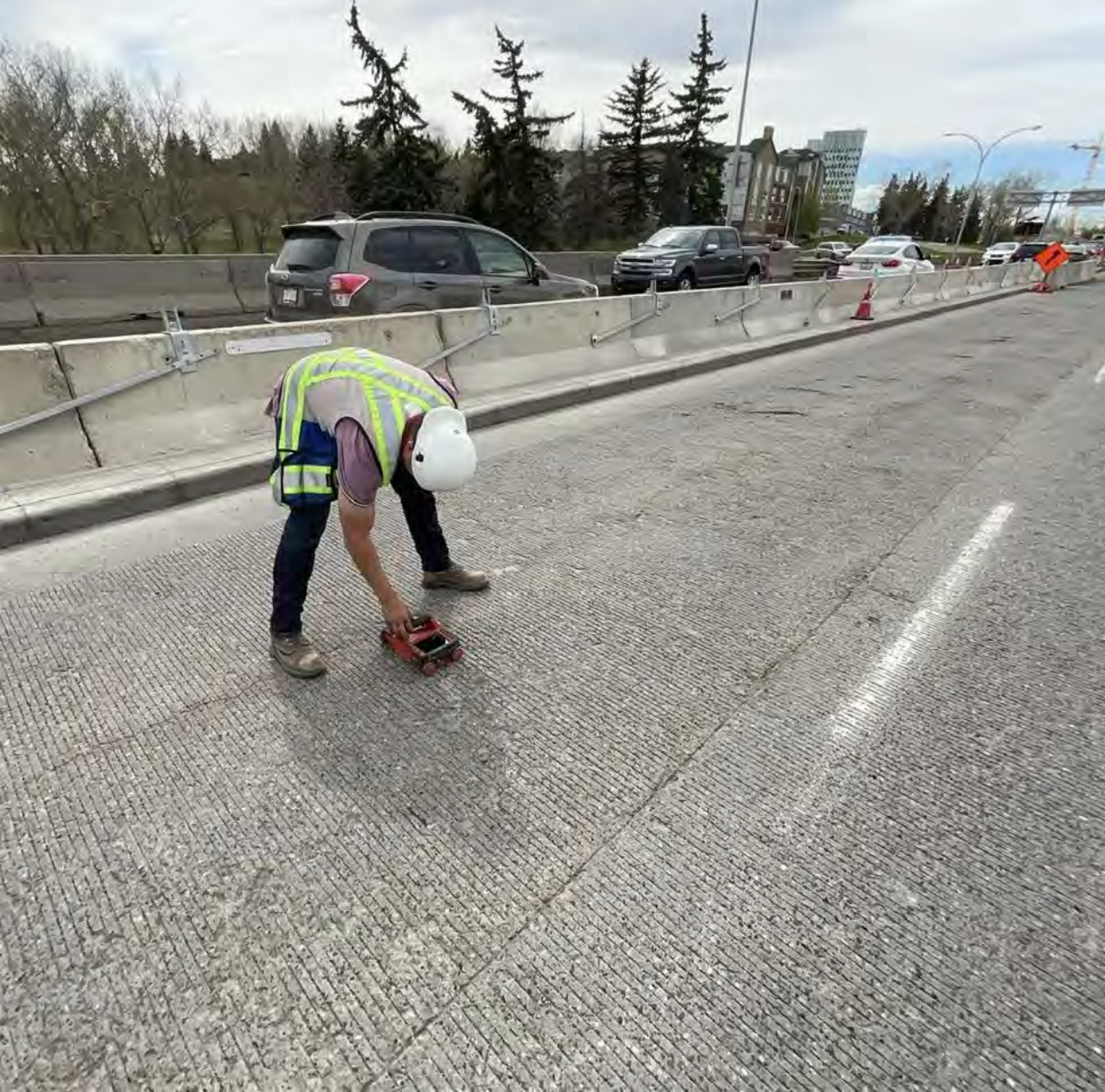
Rebar Scan and Deck Milling
