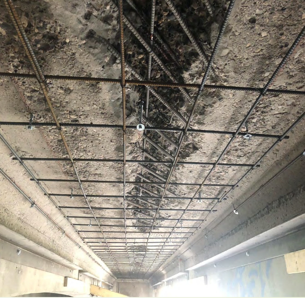
Deck Soffit and Girder Partial Depth Repairs
