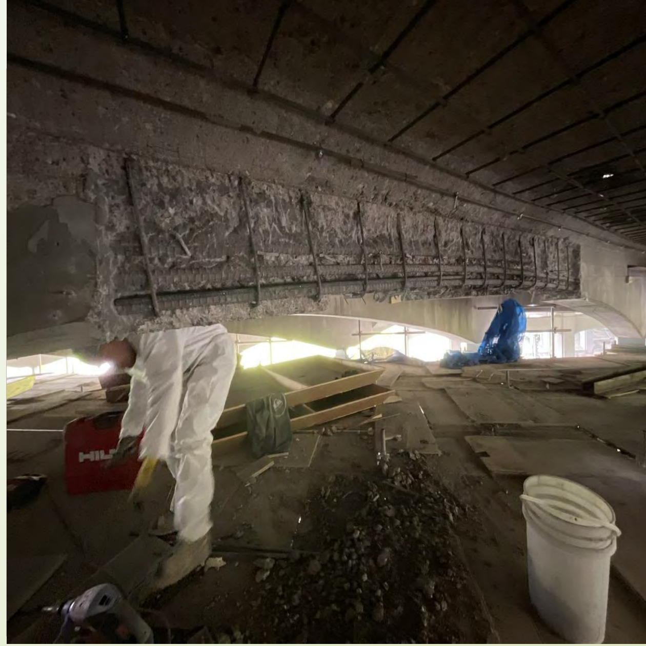
Deck Soffit and Girder Partial Depth Repairs
