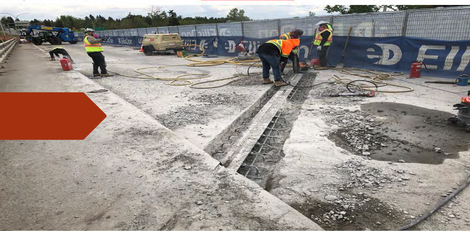
Expansion Joints Away from the abutments
